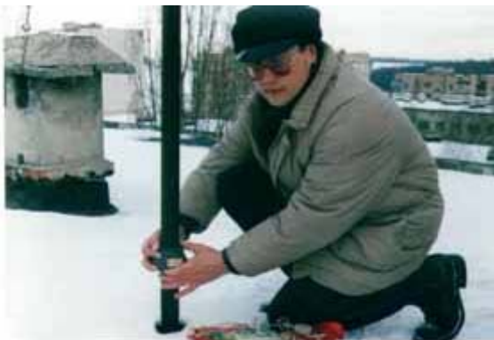
Photo: Ferrite core installed at the antenna mast base
